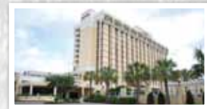
Marriott on Lockwood Boulevard in downtown Charleston.
