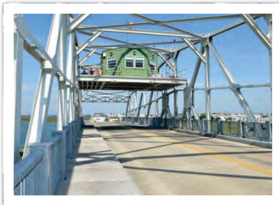
Veronica Faber's office is a green building atop the Ben Sawyer Bridge.
