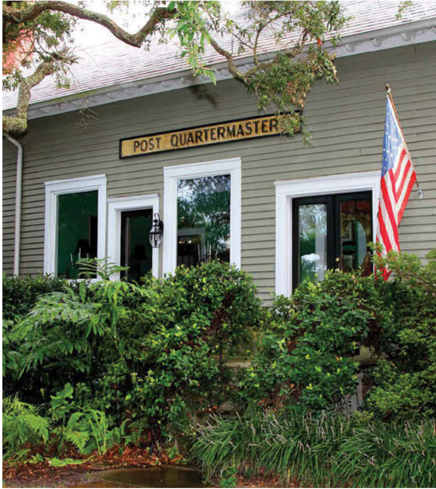
Some windows and doors have been moved since the Army days of the post quartermaster's office. The tree in front has grown, and many other shrubs and trees added over the years enhance the appearance of the building.
