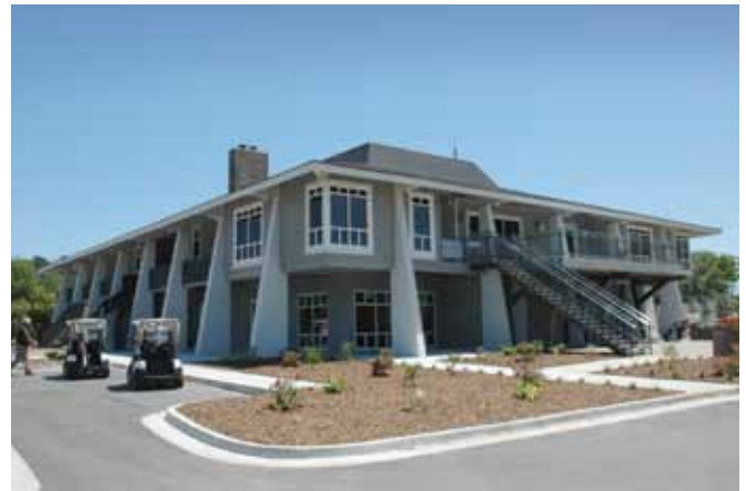
The initial plan was to demolish the old clubhouse and rebuild elsewhere. That idea was scrapped because the old clubhouse was in an ideal location, surrounded by the 18th hole, the swimming pool and the tennis courts.
