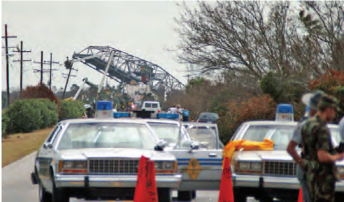
The Ben Sawyer Bridge, which connects Mount Pleasant with Sullivan's Island, was a victim of Hurricane Hugo.
